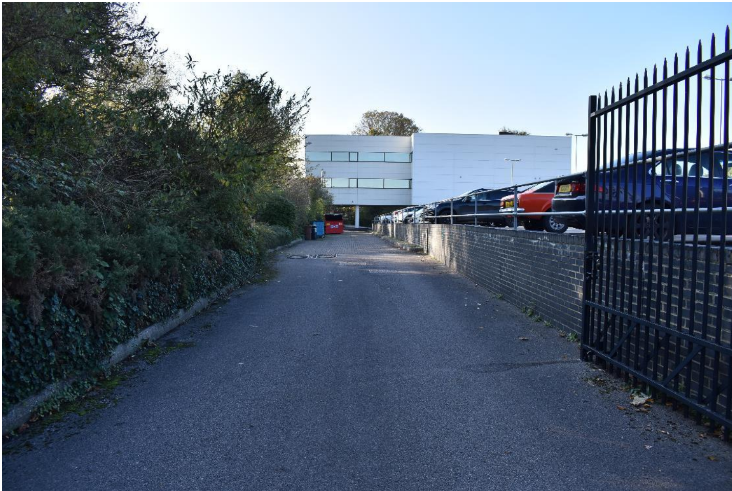
Plate 14: View along eastern boundary of the new built part of the PDA (facing SSW)
