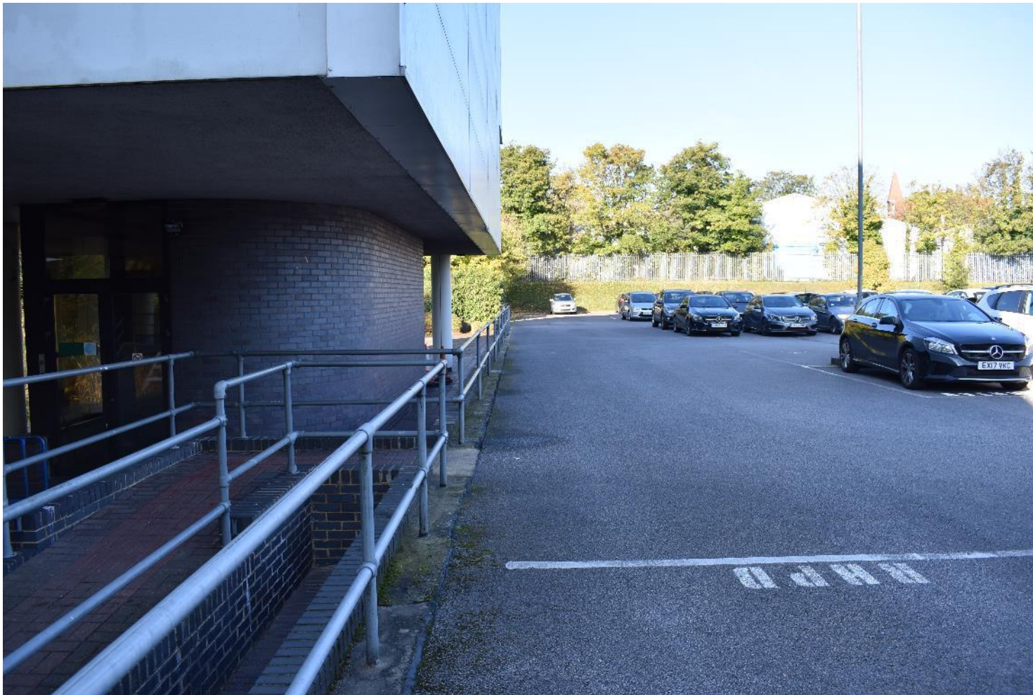
Plate 15: View along the southern boundary on the new build part of the PDA (facing WNW)
