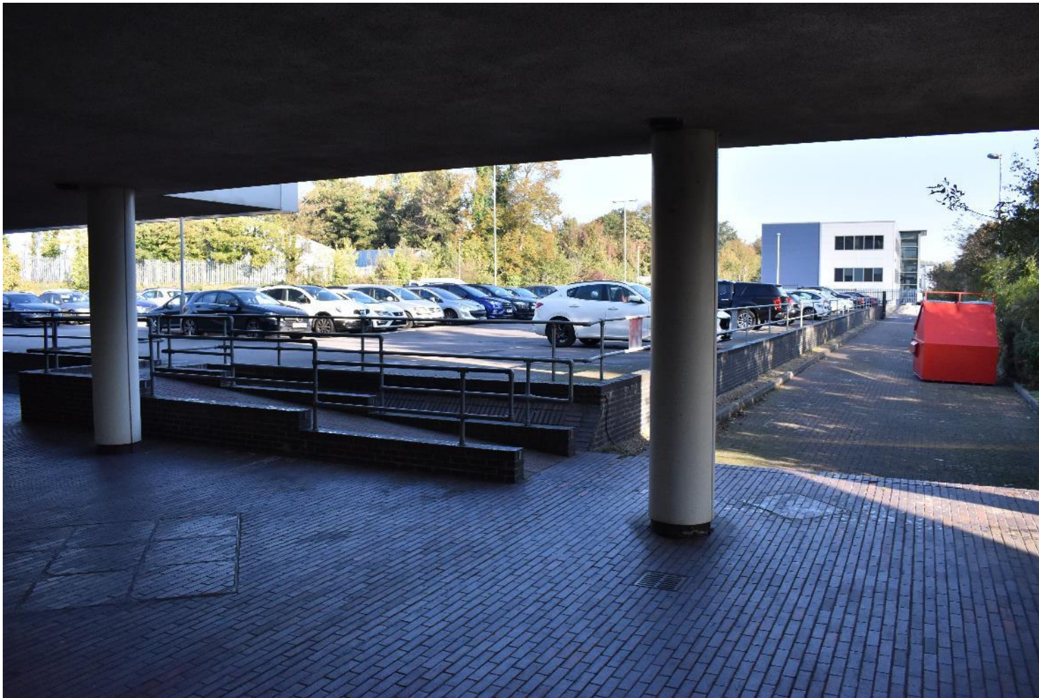
Plate 10: View across the PDA from under River House (facing N)
